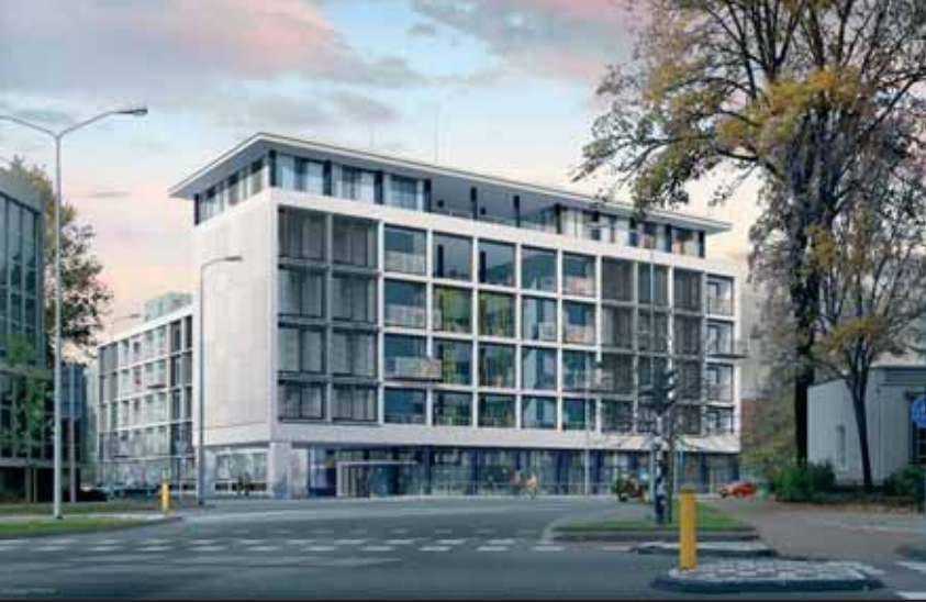
Granida (former health authority building), Eindhoven/Toon Kandelaars Architecten
