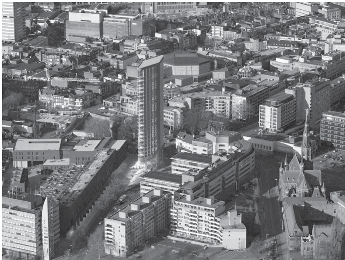
Smalle Haven project, Eindhoven
