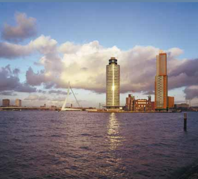
Montevideo, Wilhelminapier, Rotterdam/Mecanoo Architecten
