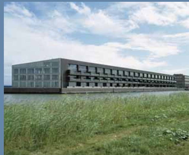
Blok 4, IJburg, Amsterdam/Maccreanor Lavington Architects
